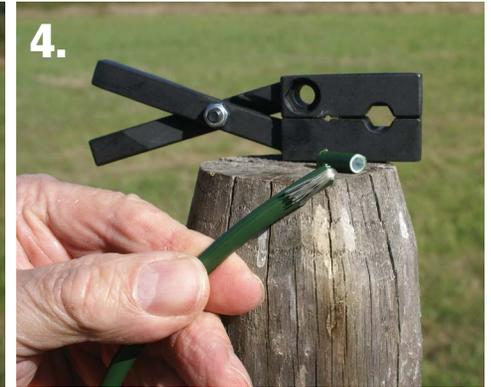
4. Bend the exposed wire back along the cable and insert into the connector
