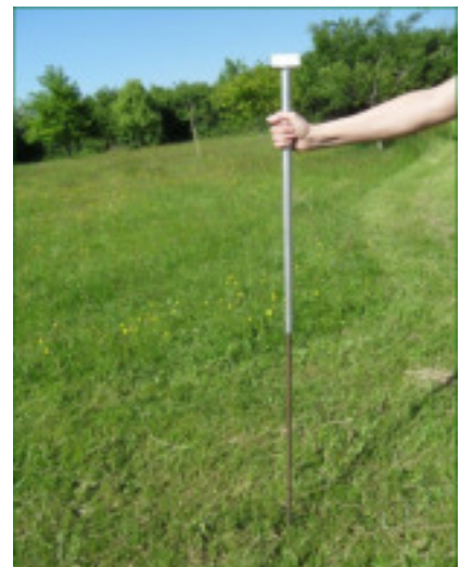
Installation of the fiberglass post with the stake driver #49
