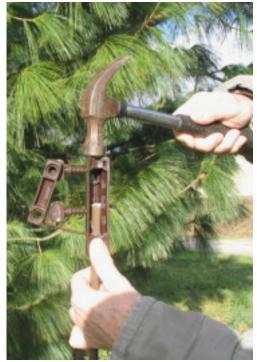
Tap firmly with a hammer on the top of the insulator until the stake passes through the precut openings on both the top and bottom of the insulator.
